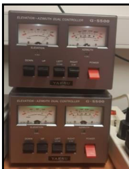
Fig. 6. Elevation-azimuth G5500 controller in the station.
